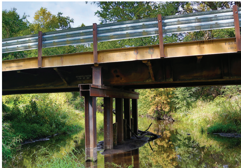
Above. Brian Keierleber says testing at Iowa State University shows that railroad flatcar bridges can support the weight of any legal load. All-steel piers offer enhanced strength and lower maintenance costs compared to reinforced concrete.
